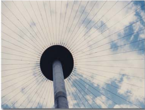
CENTER COLUMN WITH RADIAL HUB
